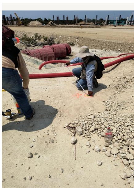
Setting out, leveling and ductwork.
